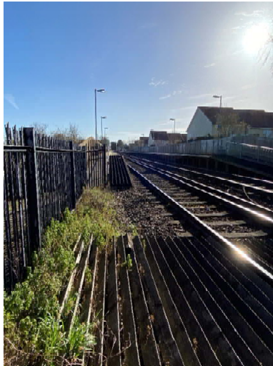
Down side up direction train approach
