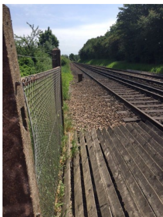
Downside up direction train approach
