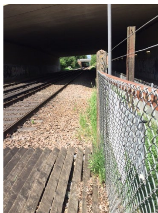
Downside down direction train approach
