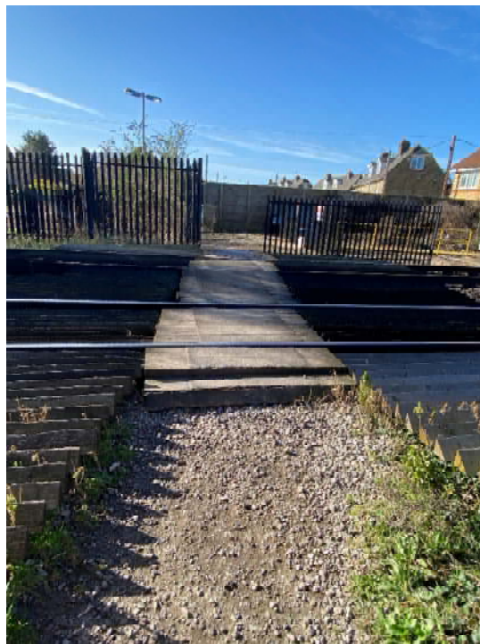
Down side across crossing
